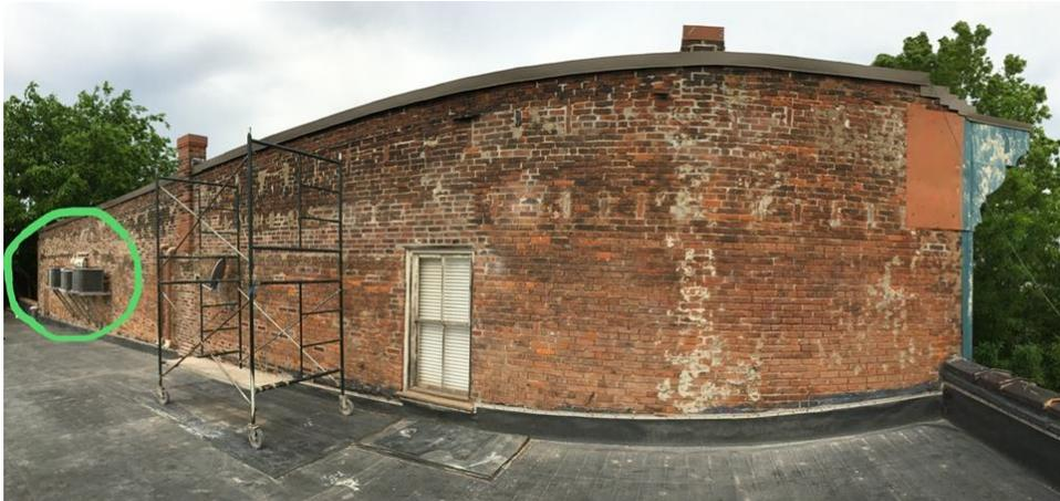
*Locate mechanical systems on rear elevations or behind parapet walls on the roof. No systems should be visible from the public right of way.*
