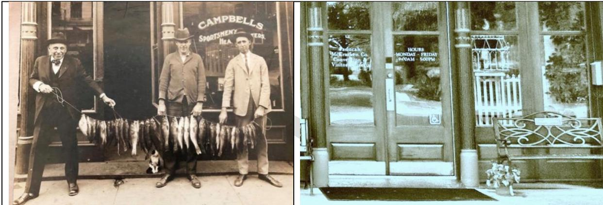
*128 Broadway - an example of pictorial research to determine original or early design of a storefront. It would be optimal if the original right window were still intact. Keeping the materials and designs that are still intact—cast iron columns, sills, and bulkhead design—reflect proper treatment.*
