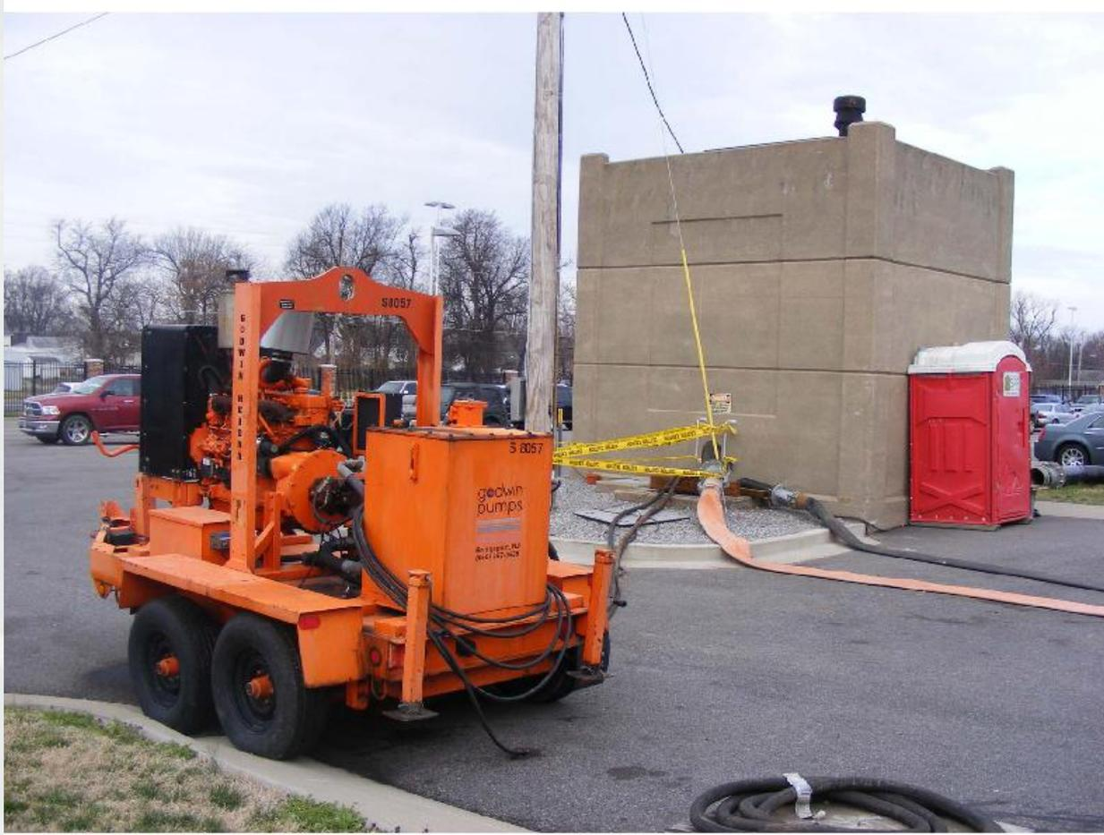
PS#9, Pump Temporary Pumps added to the station to offset lost pumping capacity at this station.
