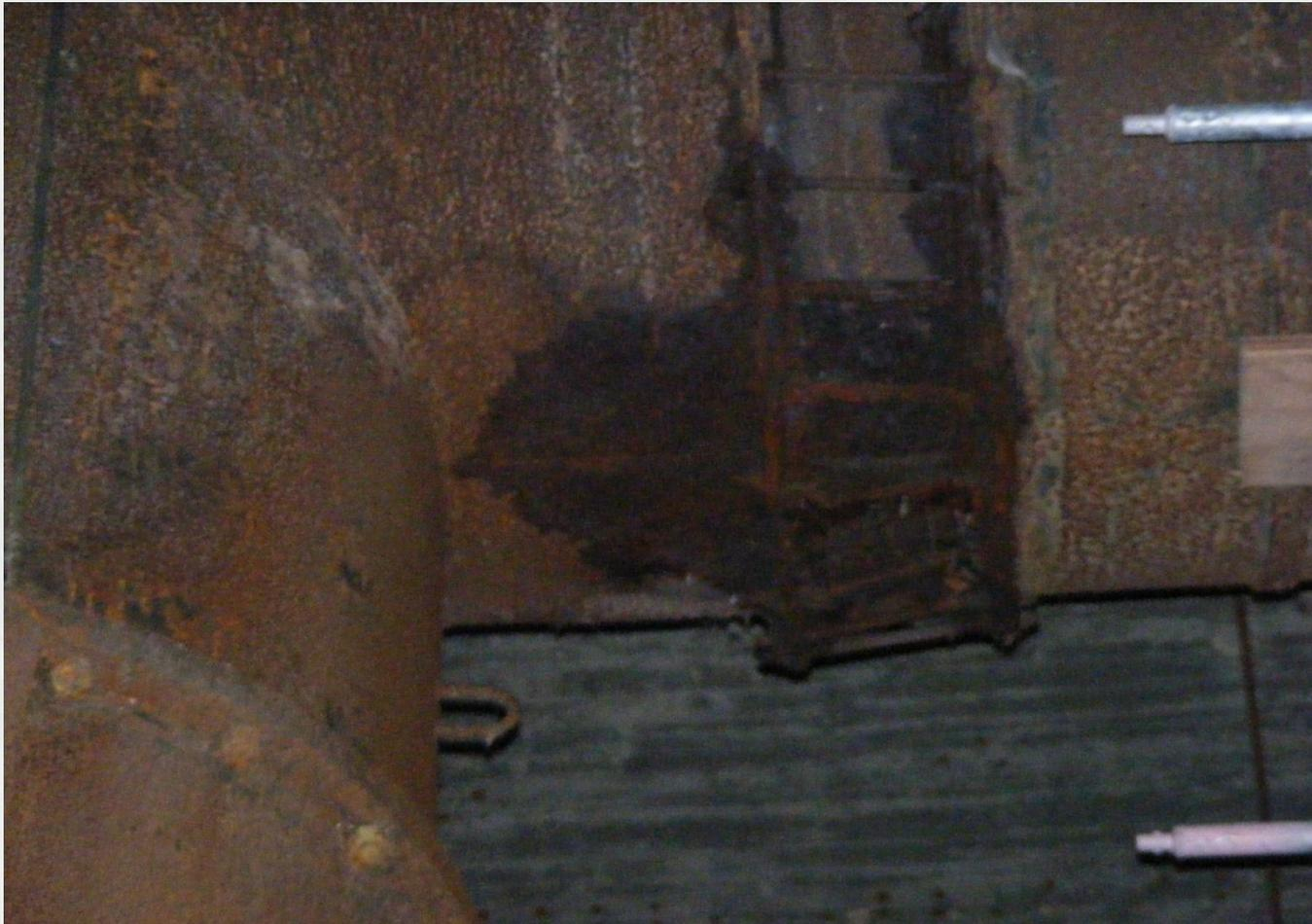
PS#2 discharge pipe coupling ruptured.
